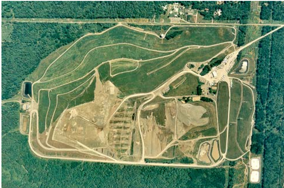
Aerial View of Cedar Hills Landfill – May 1998
